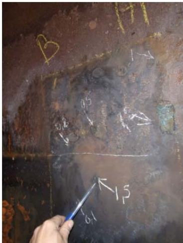
Localised pitting corrosion. Min. wall thickness above/below waterline: 50.3 / 48.7mm. Average: 51.0 mm => Max variation: 0.7/2.3 mm.
